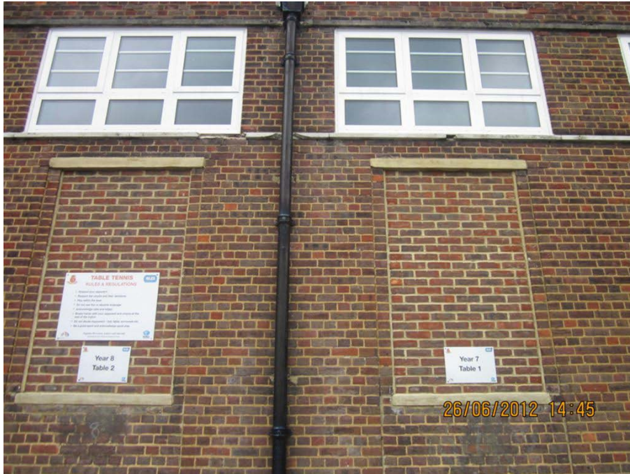
Figure 3- Defective Concrete Structural Elements
