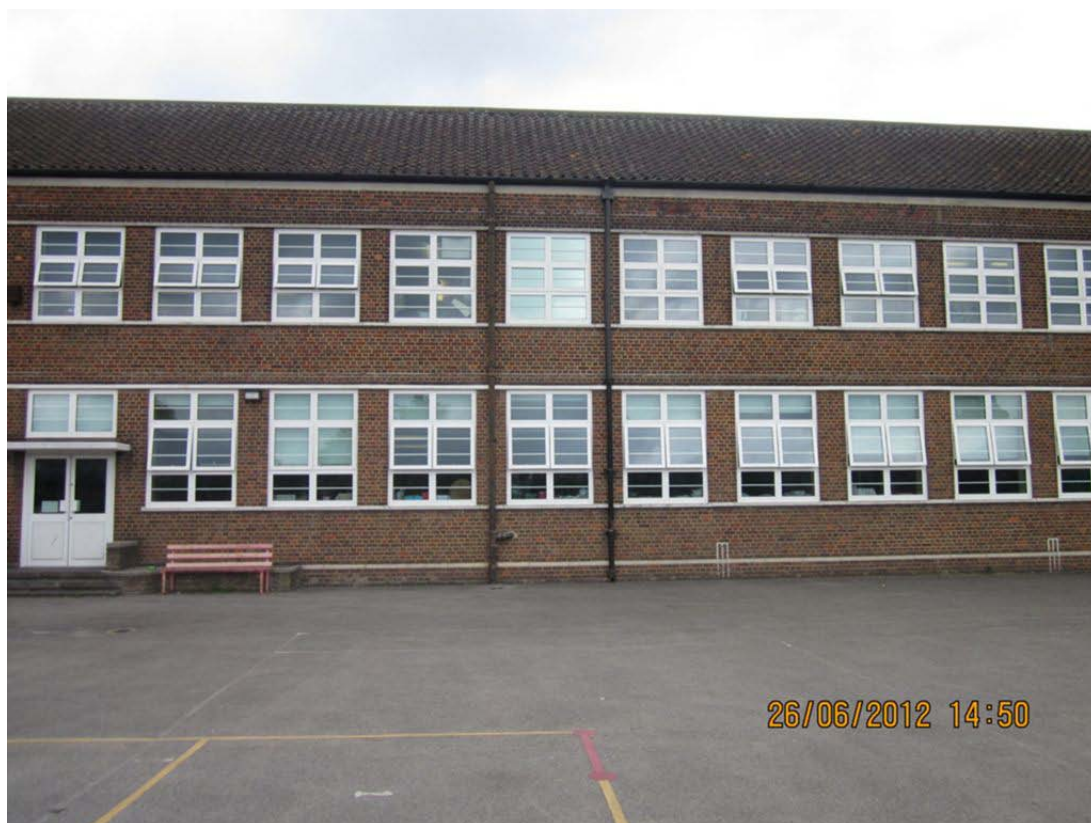
Figure 1- Exterior of Block A
