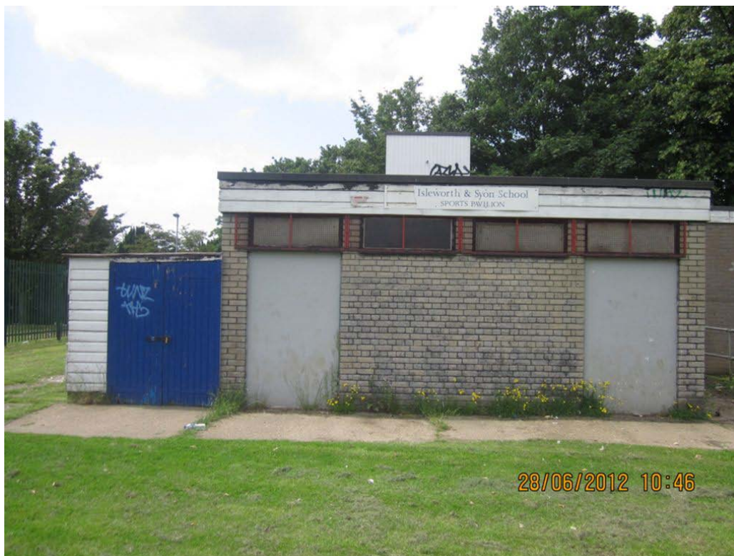
Figure 7- Exterior of Block C
