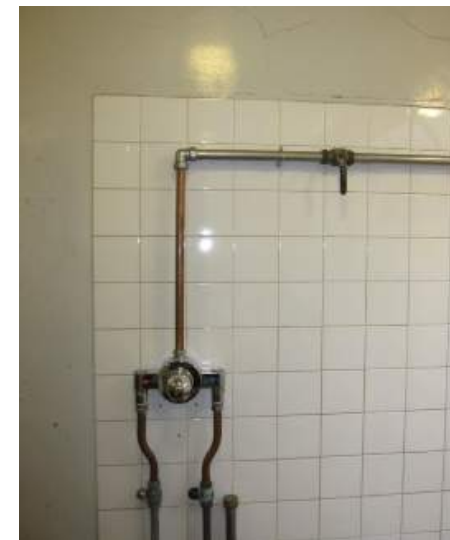
Figure 3.17 - Single Ball-o-Fix isolating valve serving all shower outlets
