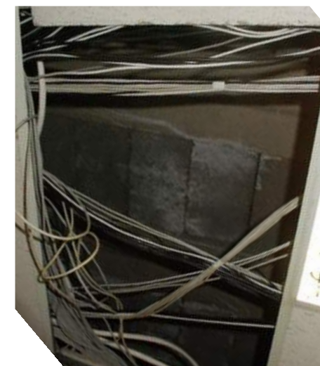
Figure 3.2 - Exposed roof construction in the IT room (no insulation)
