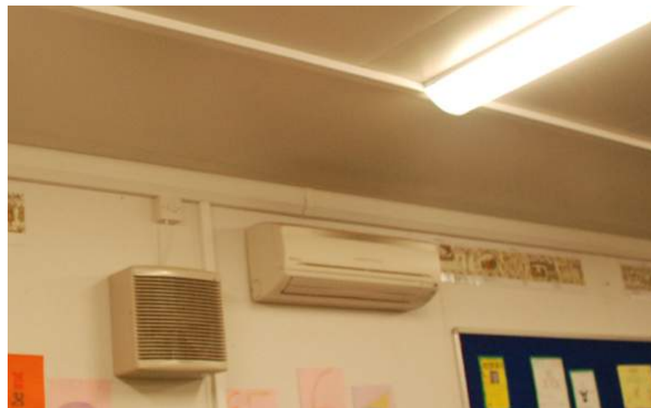
Figure 3.15 - Extract fan and cooling unit in the teaching huts.
