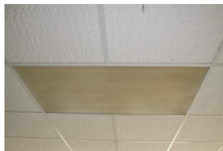
Figure 3.18 - Photo-degraded (yellowed) light diffuser (one of many)
