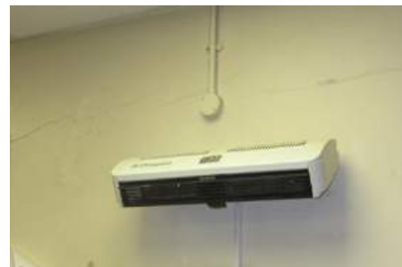
Figure 3.10 - Resistance heaters
