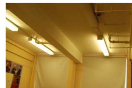
Figure 3.19 - Linear fluorescents behind acrylic diffusers with poor light output (one of many)
