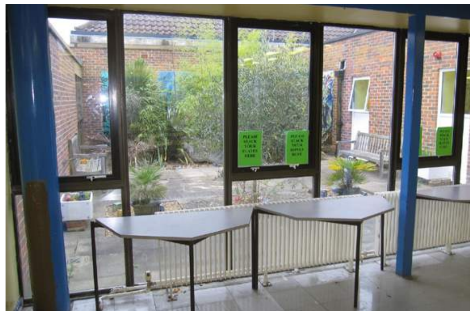
Figure 3.3 - Full-height single-glazing in the Canteen – the lower third contributes negligible daylight but suffers very high heat loss
