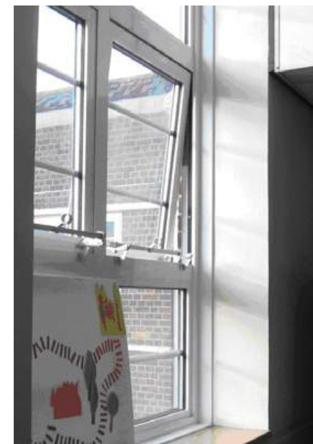
Figure 3.1 - Typical replacement double-glazed window, hinged at the top)
