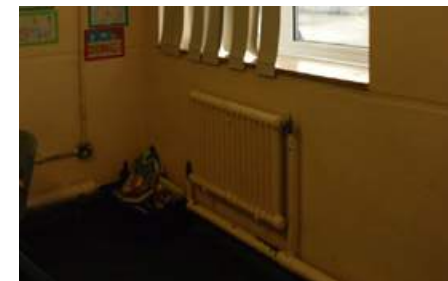
Figure 3.5 - Typical radiator detail with no control
