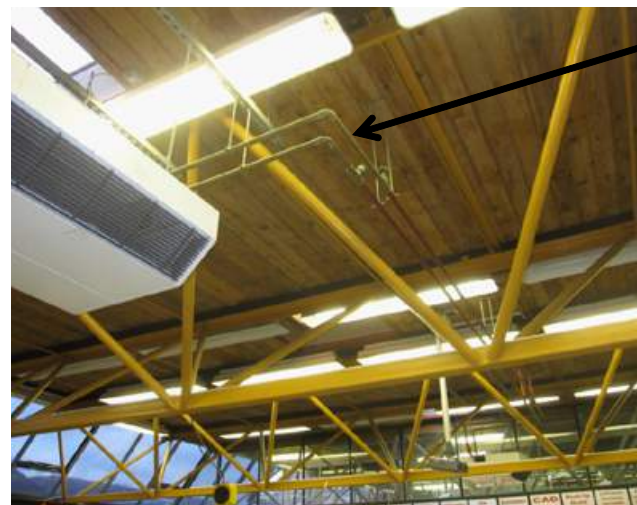
Figure 3.9 - Exposed heating pipework, releasing heat above the occupied zone and without control
