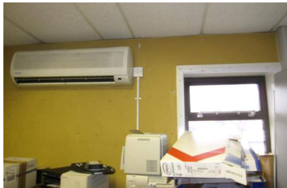
Figure 3.14 - Manufactured ‘cold air’ to the left, and unused free cold air to the right.
