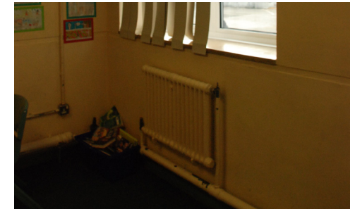
Figure 2.5 - Typical radiator detail with no control
