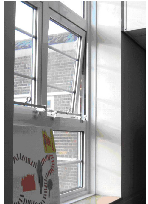
Figure 2.1 - Typical replacement double-glazed window, hinged at the top)
