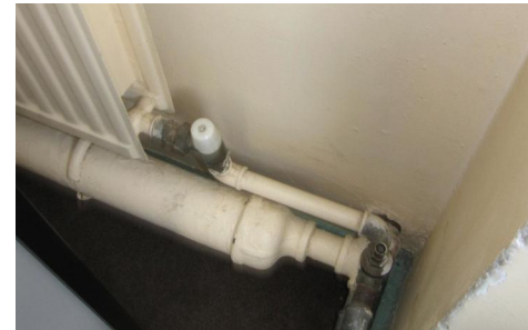
Figure 2.4 - Typical radiator detail with no control, and very large diameter pipework for gravity circulation (loses lots of heat)
