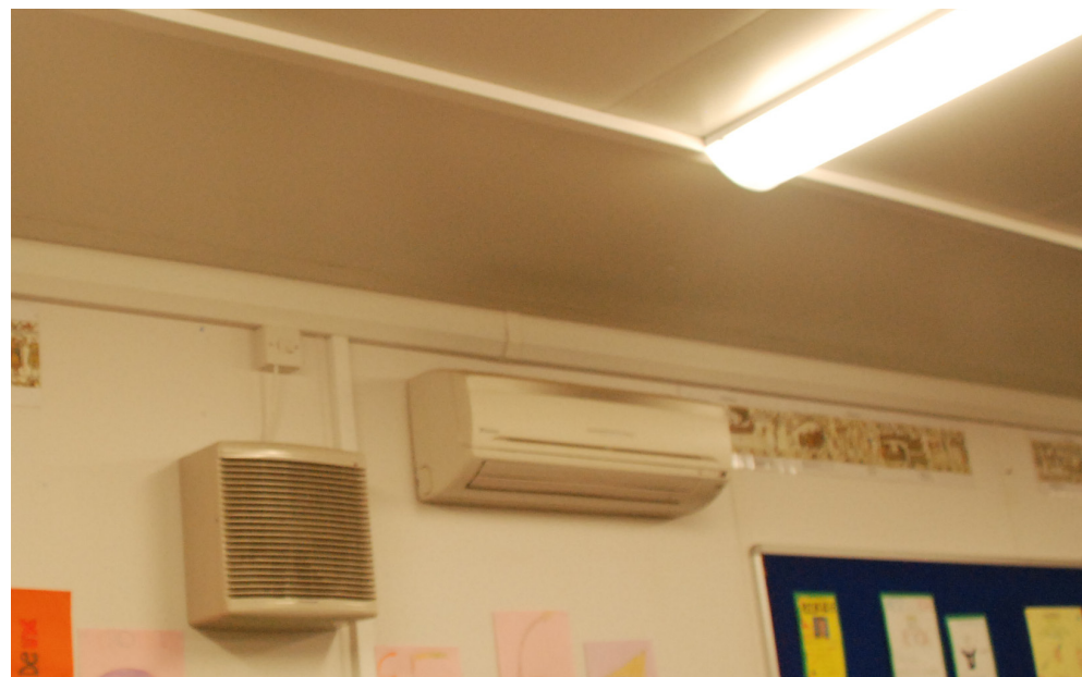
Figure 2.15 - Extract fan and cooling unit in the teaching huts.
