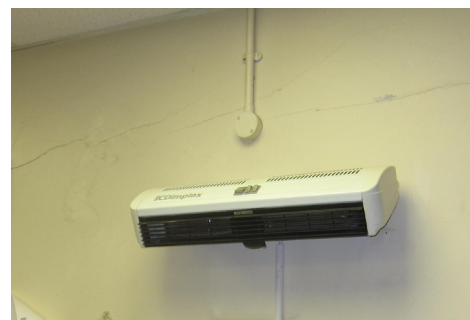
Figure 2.10 - Resistance heaters
