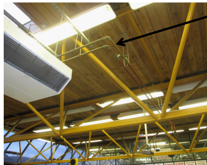
Figure 2.9 - Exposed heating pipework, releasing heat above the occupied zone and without control
