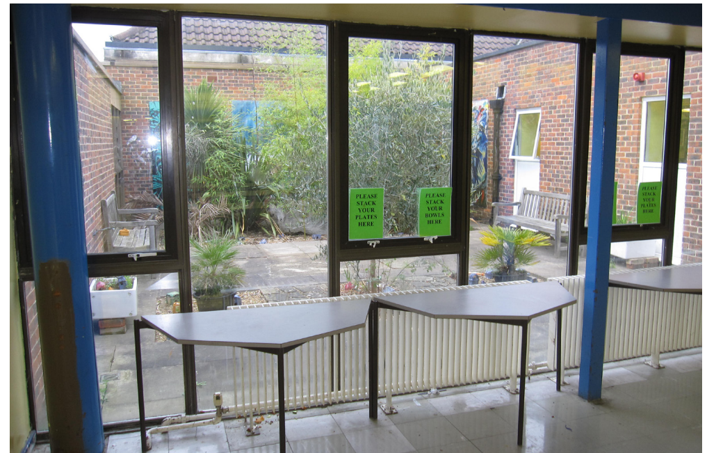
Figure 2.3 - Full-height single-glazing in the Canteen – the lower third contributes negligible daylight but suffers very high heat loss
