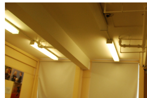
Figure 2.19 - Linear fluorescents behind acrylic diffusers with poor light output (one of many)
