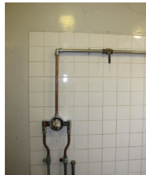
Figure 2.17 - Single Ball-o-Fix isolating valve serving all shower outlets
