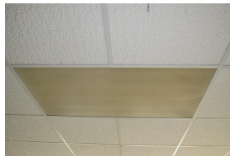
Figure 2.18 - Photo-degraded (yellowed) light diffuser (one of many)
